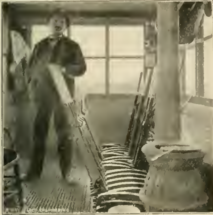
INTERIOR OF INTERLOCKING TOWER ON PASSAIC BRIDGE—D, L. & W.
